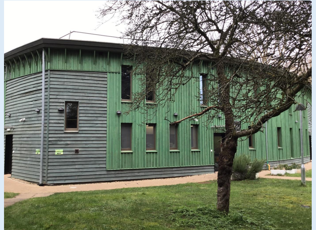
The Ark (Dining room, meeting rooms and accommodation)
